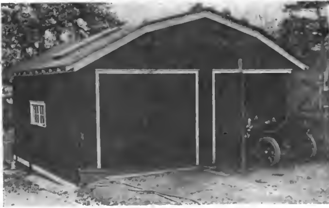
Garage Which Was Stretched from One to Two Cars' Capacity
